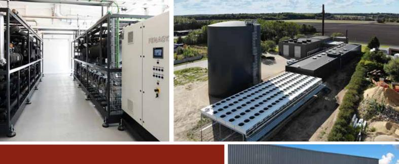
YEAR: 2022 MODEL: 2 X H-1800 (AW) APPLICATION: Air-to-water heat pump CAPACITY (HEAT): 3.5 MW (0°C ambient, 35/70°C hot water) COP: 2.96 DEFROST METHOD: Glycol
